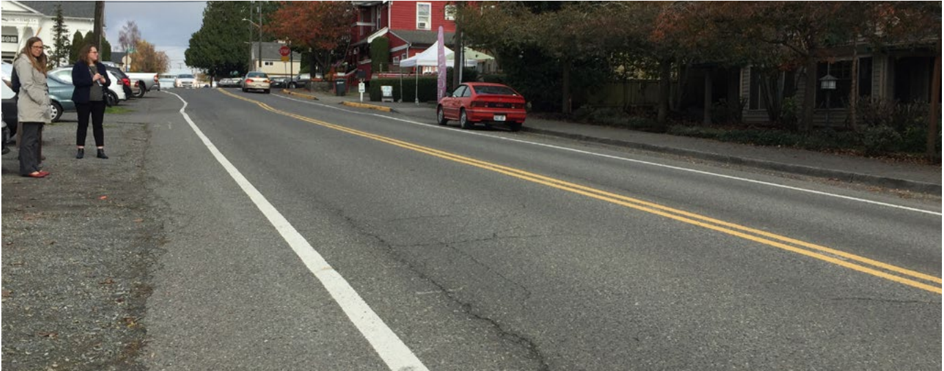
Above: Narrow street shoulder and lack of sidewalk along 10th Ave.
