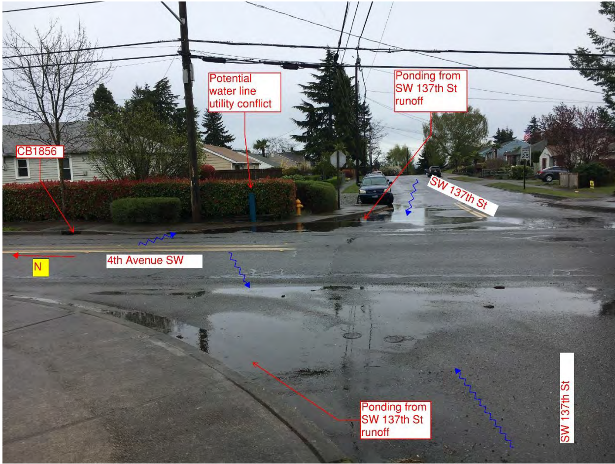
FIGURE 2: Ponding at NE and NW corner of SW 137th Street and 4th Avenue SW. Photo date 4/8/2019
