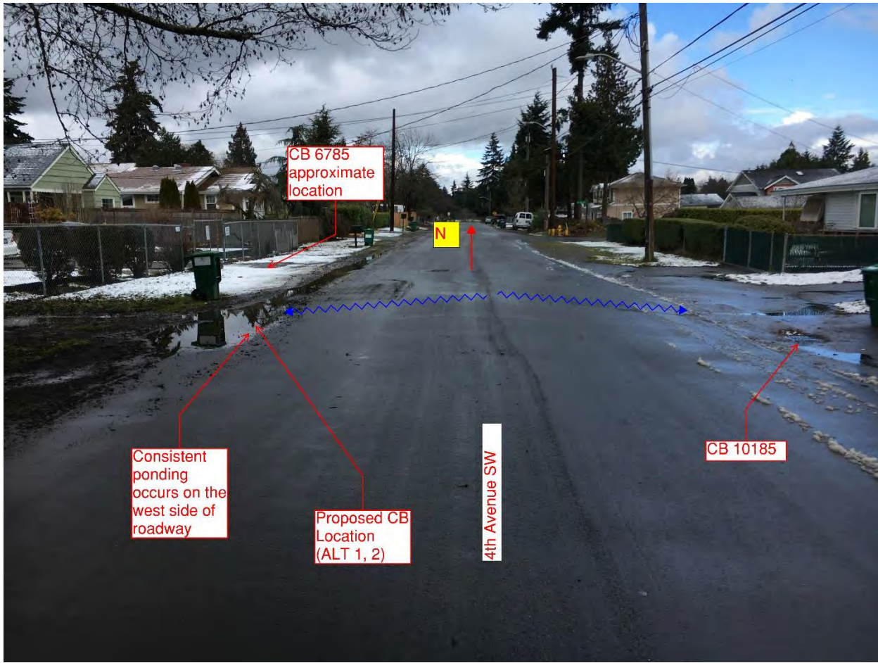
FIGURE 1: Ponding on 4th Avenue S, facing north. Photo date 3/7/2019
